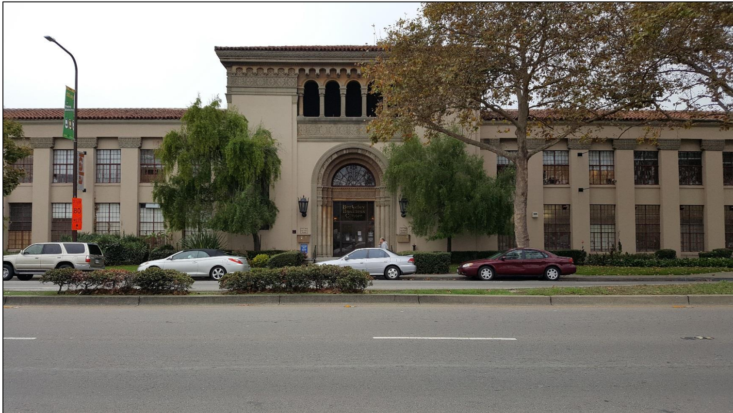
Historic Heinz Building, San Pablo and Ashby
